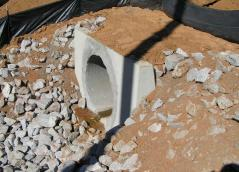
Use **Pipe Straight Headwall** (719-605-00) when specified in the plans or special provisions. Use straight headwall only in locations where pipe exposed end does not face the direction of traffic.
